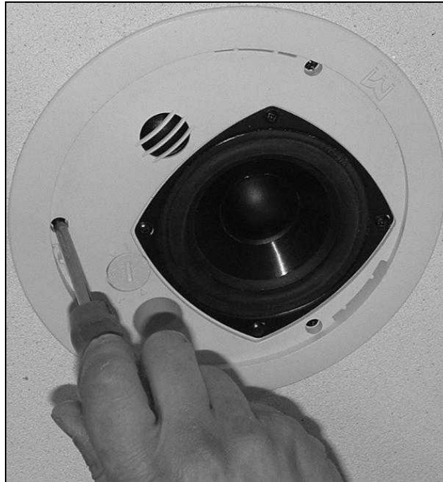
Tightening the swivel-tab screws
